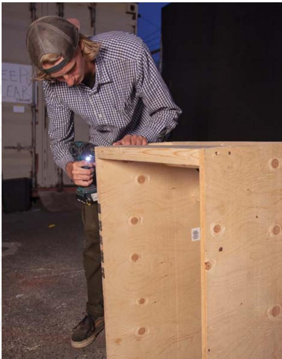
**4.** Go back and add a second screw on all the ribs, on both sides of the transition and the supporting ribs, double checking that each rib is flush.
